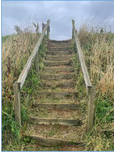
steps cleared of vegetation by a volunteer
